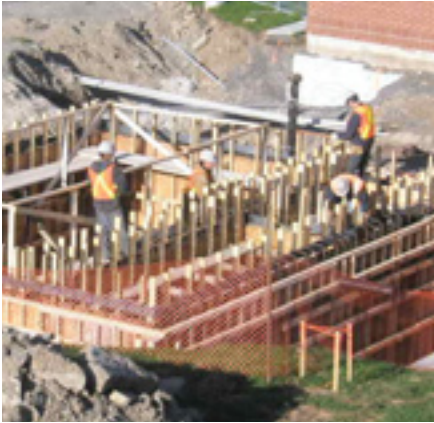
Tank construction for the dewatering facility upgrade
