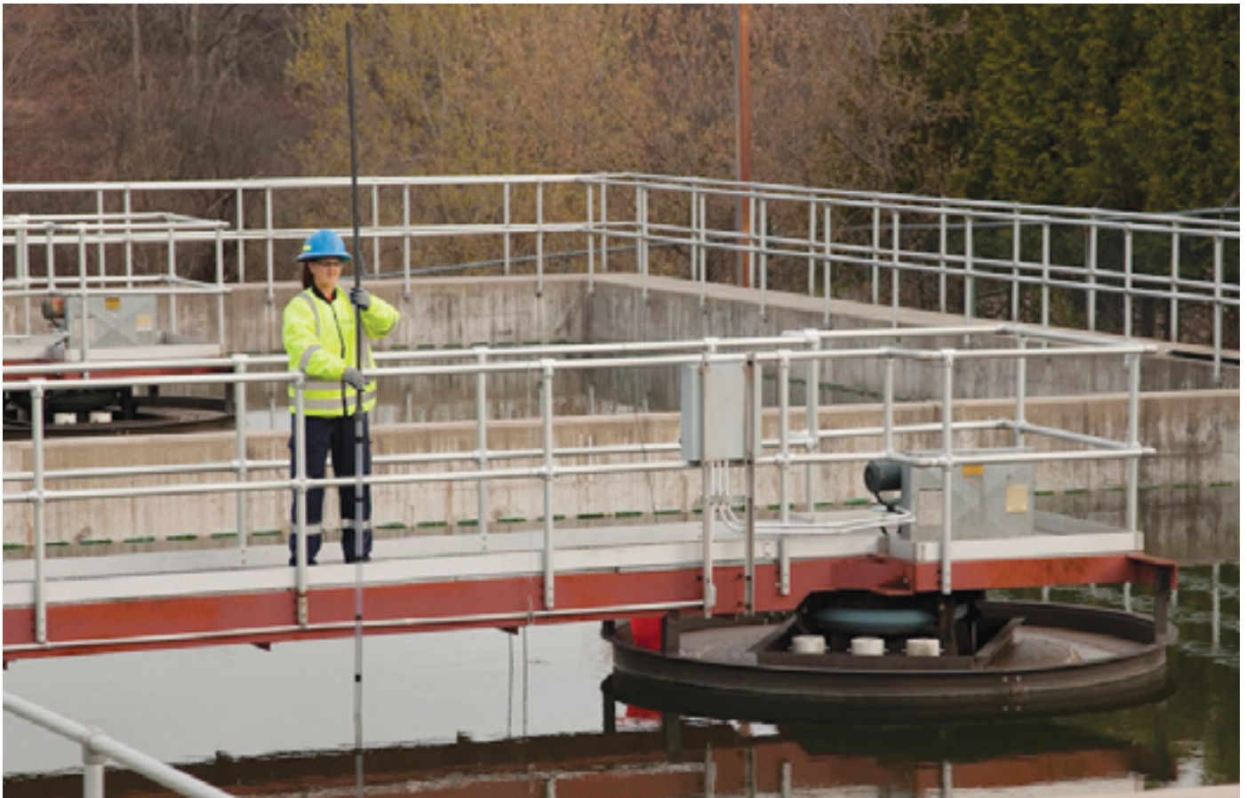
Operator Mandi Larose performs routine checks and sampling at WWTP
