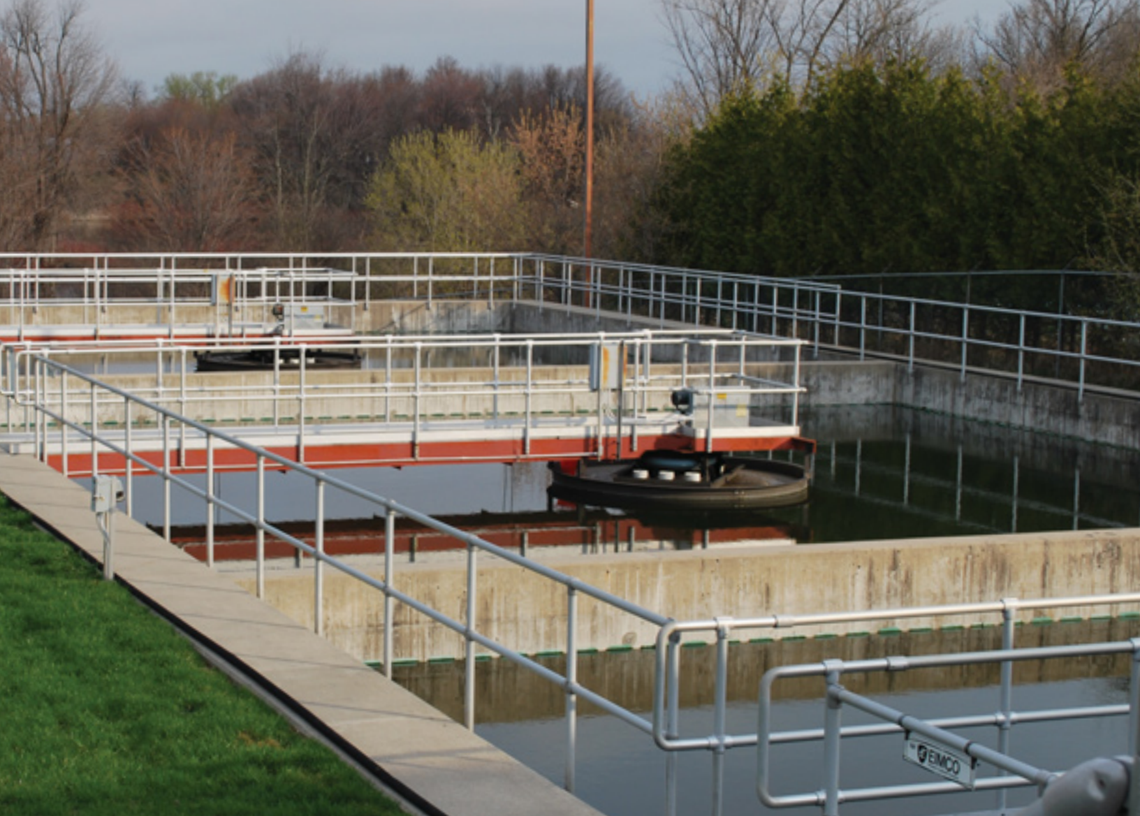
Wastewater Treatment Plant secondary clarifiers
