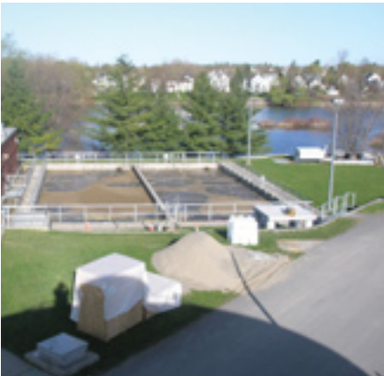
Aerial view of aeration tanks
